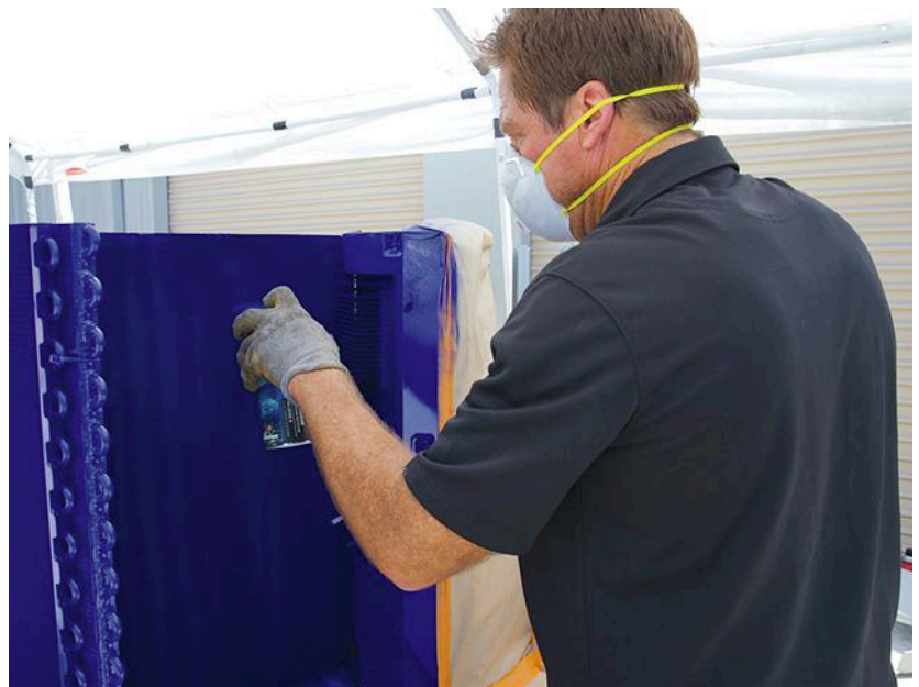
Some coatings are blue so the applicator can visibly track even coverage of the sprayed area.
