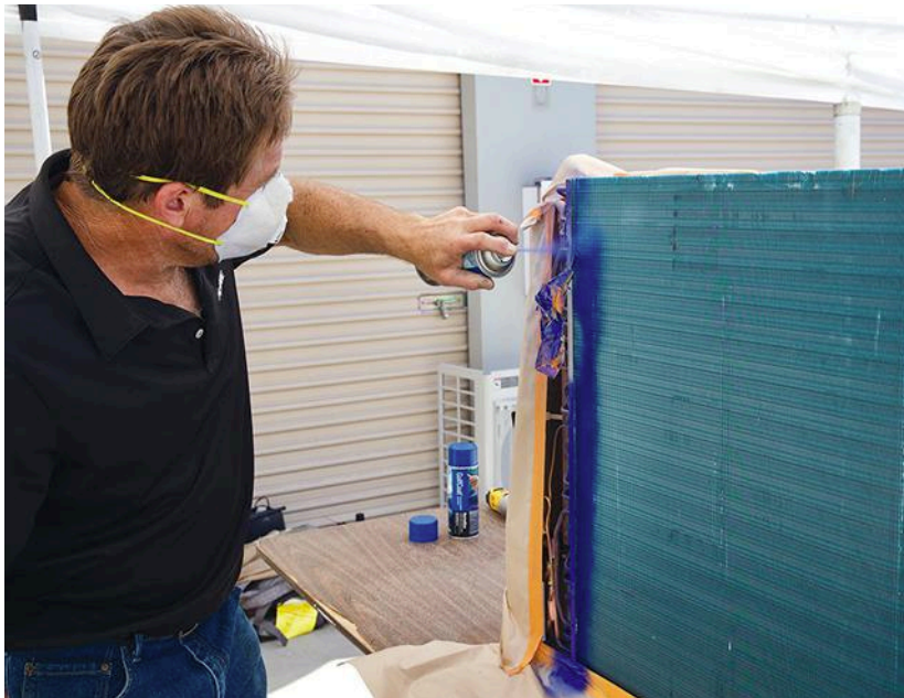
DIY: Contractors can spray the coil coatings, themselves, saving the time and money involved in outsourcing the work to a factory.
