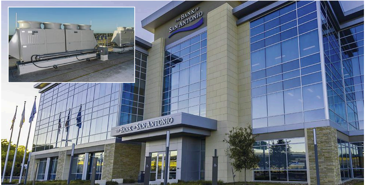
Zone control: In 2015, the Bank of San Antonio built a new, 56,000-sq-ft branch and office facility downtown. Needing to find an energy-efficient HVAC system, the owner chose a rooftop VRF unit (inset) that has provided quality comfort with flexible control.
