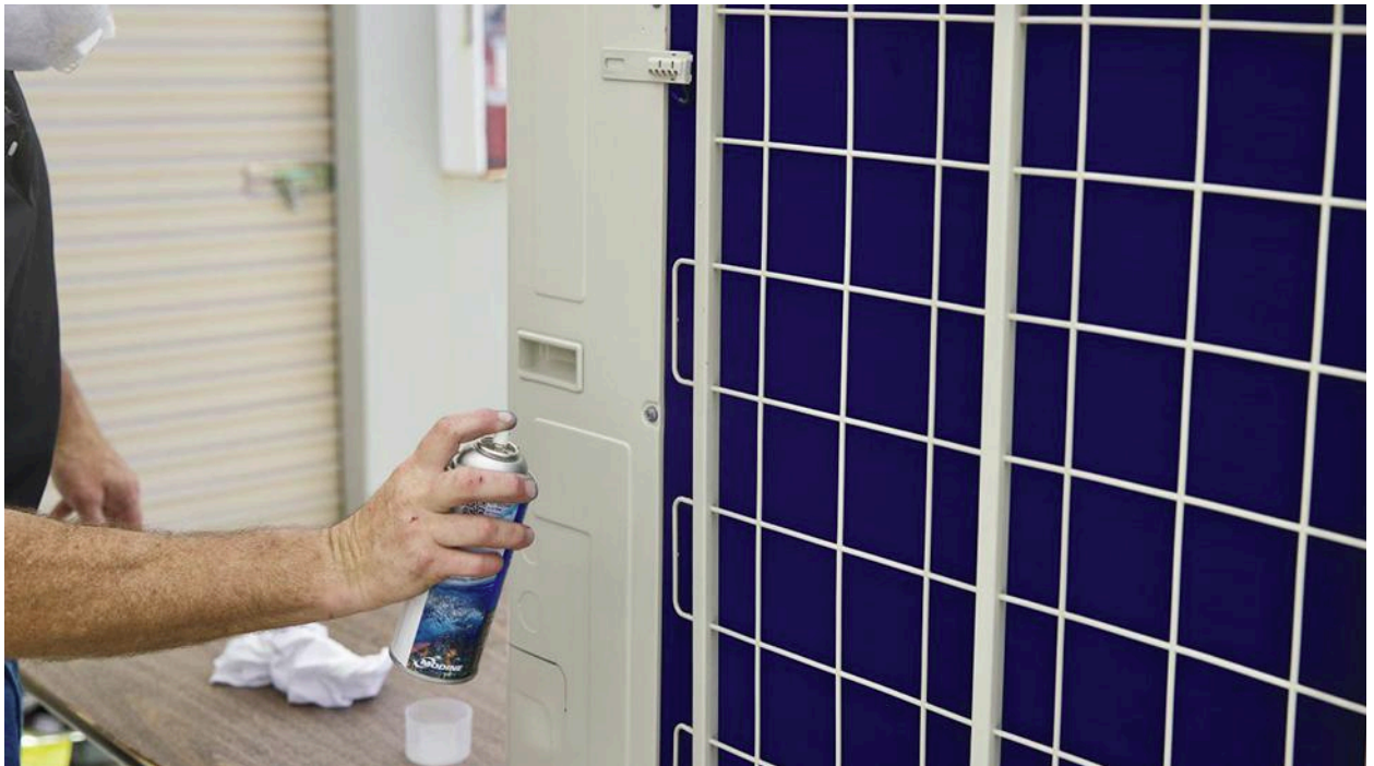
Contractors can now coat coils in their shop or onsite before installation with coatings packaged in convenient aerosol cans.
