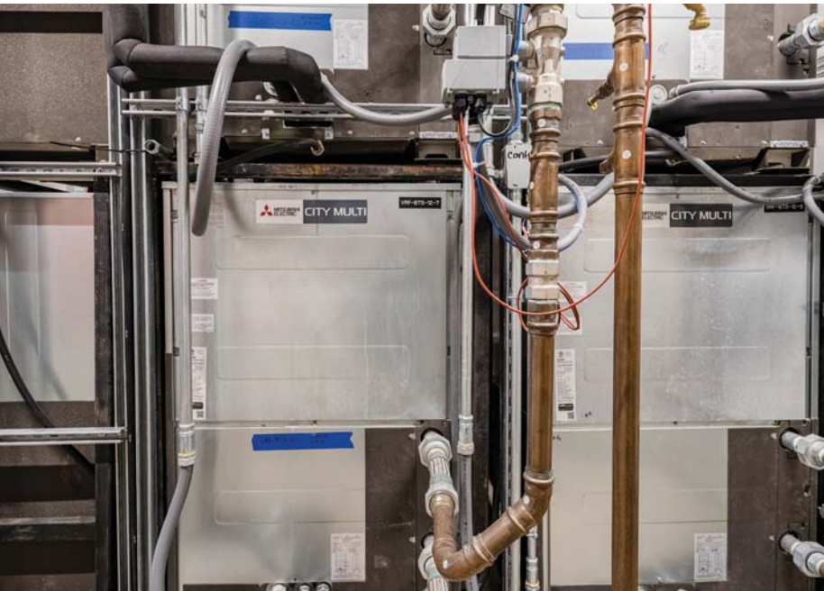
All of the equipment in a ground-linked water-source VRF system is designed to be installed indoors.
