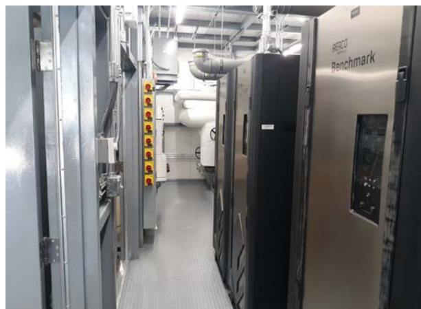
Since installation, overall boiler efficiency has greatly improved while maintenance needs have gone down.
