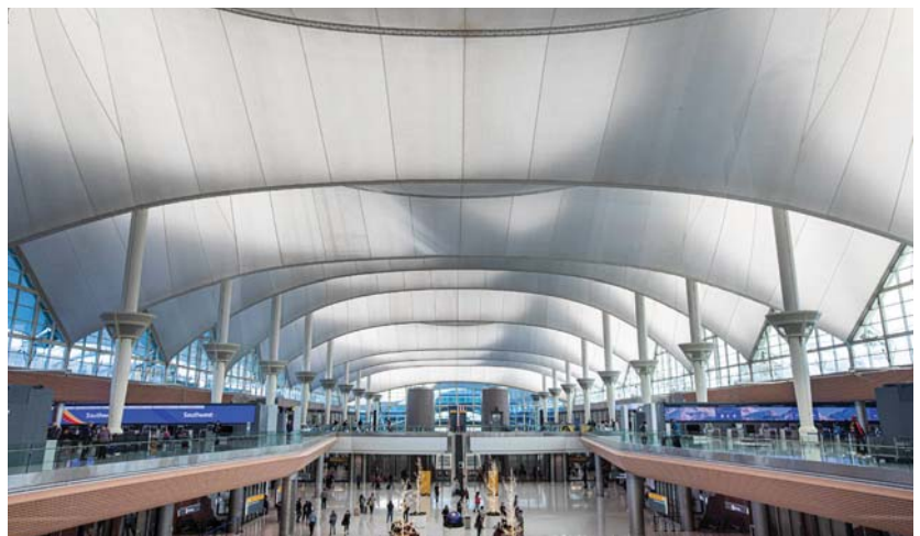
Denver's massive airport utilizes an impressive battery of hot water boilers.
